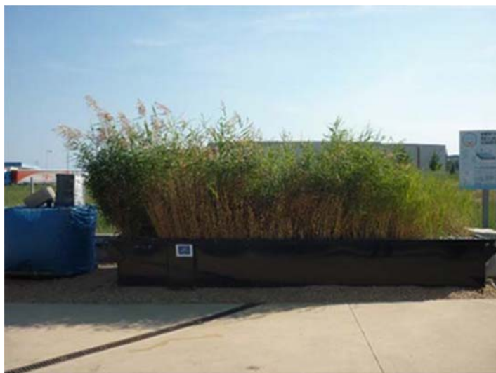
Figure 21.5 View of the pilot HFCW.
